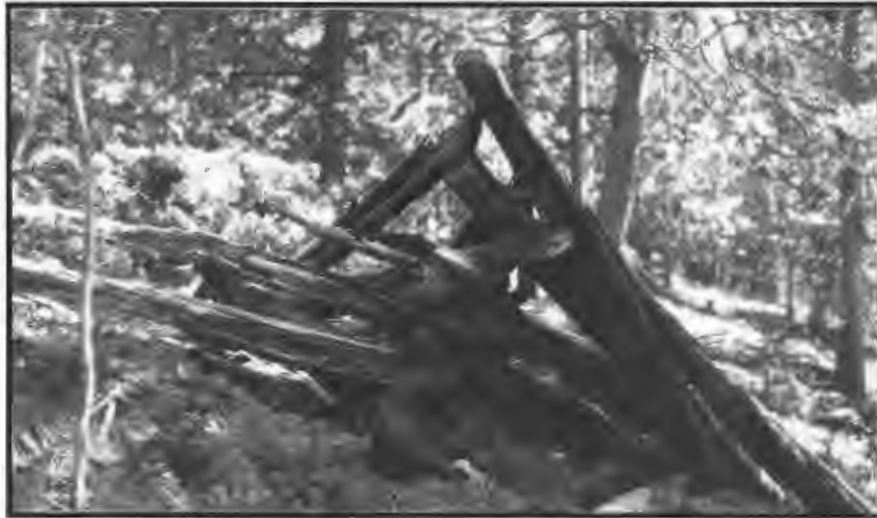
Figure 32. Collapsed remains of Feature 68 residence at south end of 24BW210.
