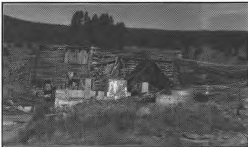
Figure 9. Feature 37 mill foundation and associated ore bin.
