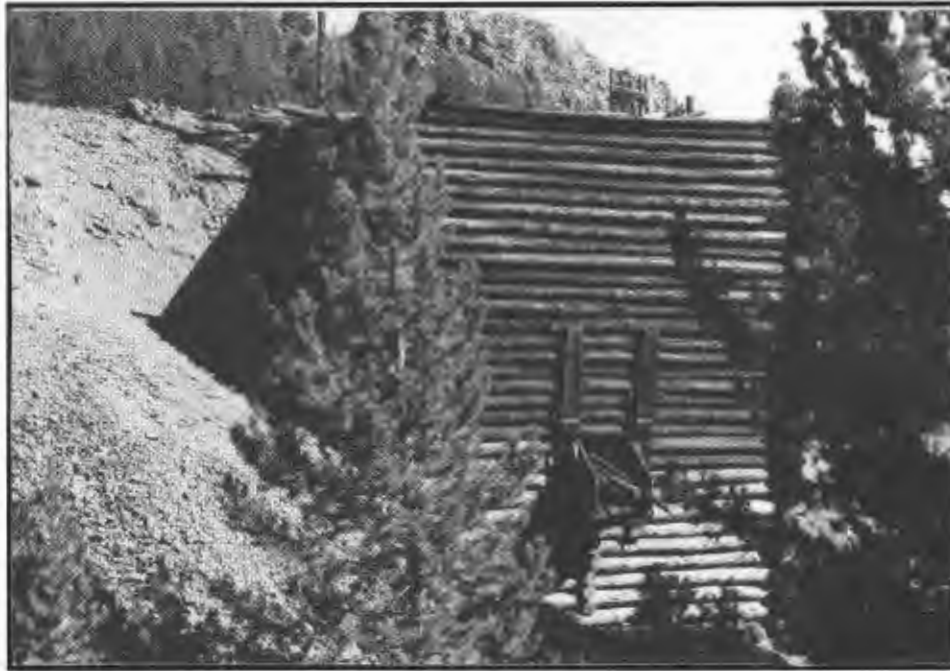
Figure 6. Ore bin at Feature 8, near center of 24BW210.
