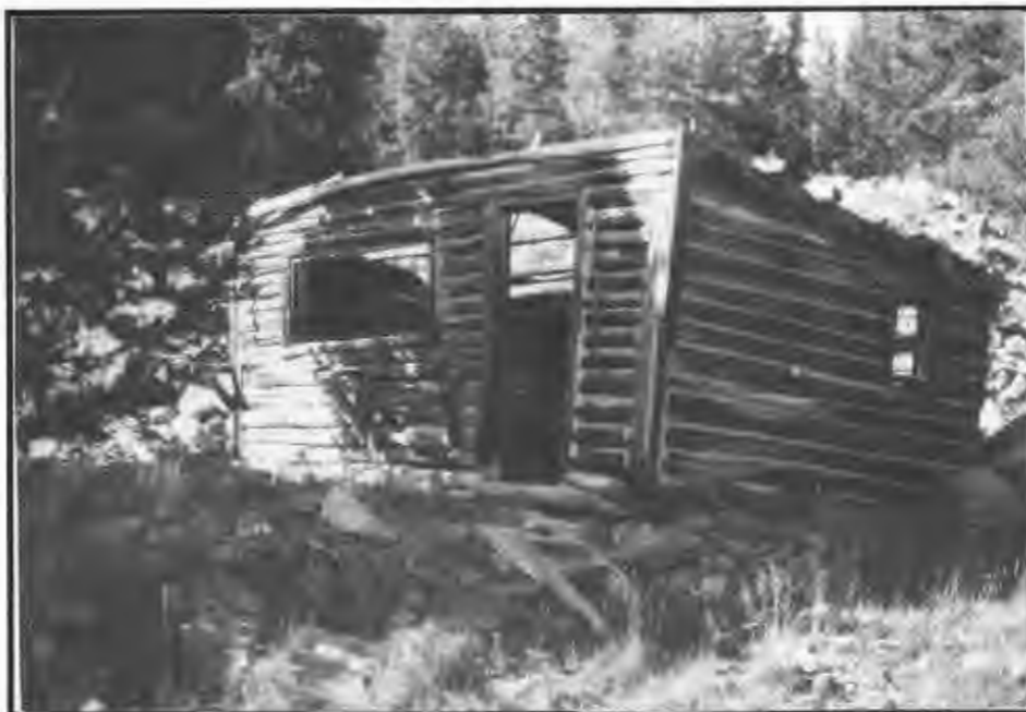
Figure 13. Feature 25 shop at base of Feature 23 waste rock pile, near center of 24BW210.
