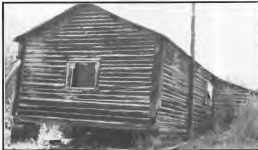
Figure 25. Rear and side of Feature 50 residence, showing cinder block footings.
