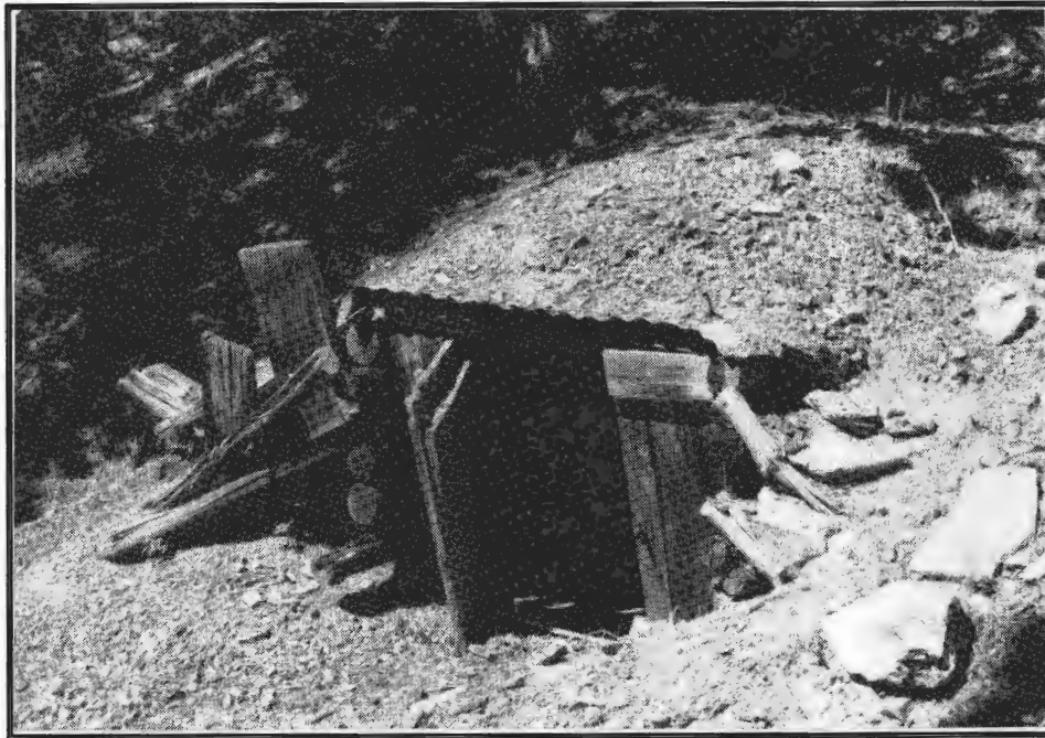
Figure 16. Feature 19 powder magazine excavated into waste rock pile.
