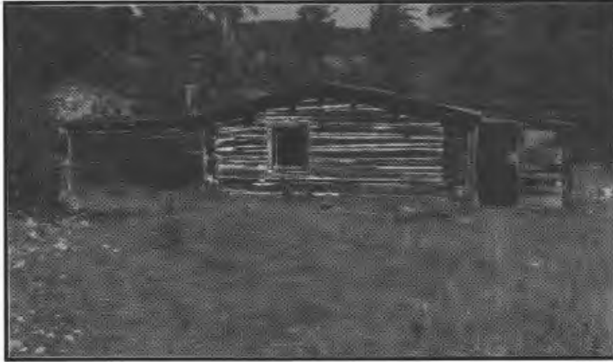
Figure 31. Side of Feature 62 residence, showing original room (center).
