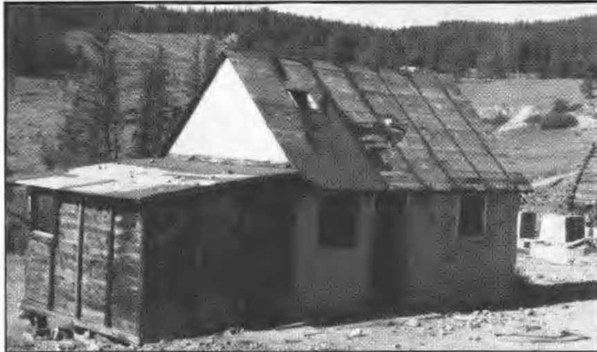
Figure 20. Feature 63 assay office, with Feature 37 mill in right background.
