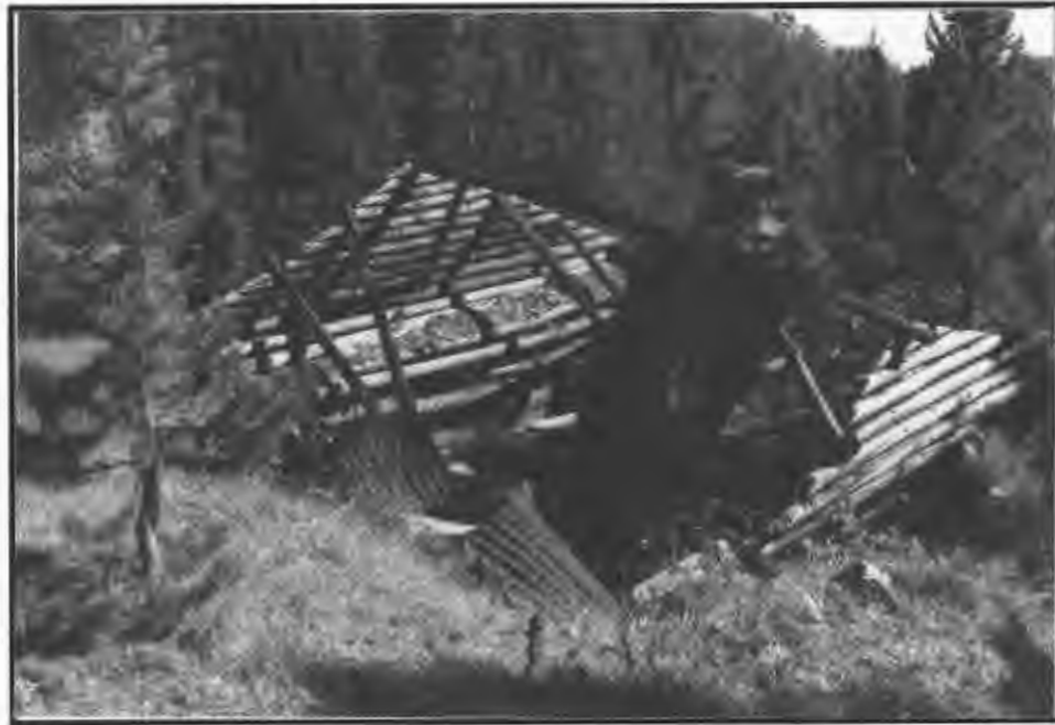
Figure 34. Partially collapsed Feature 15 at center of 24BW210.
