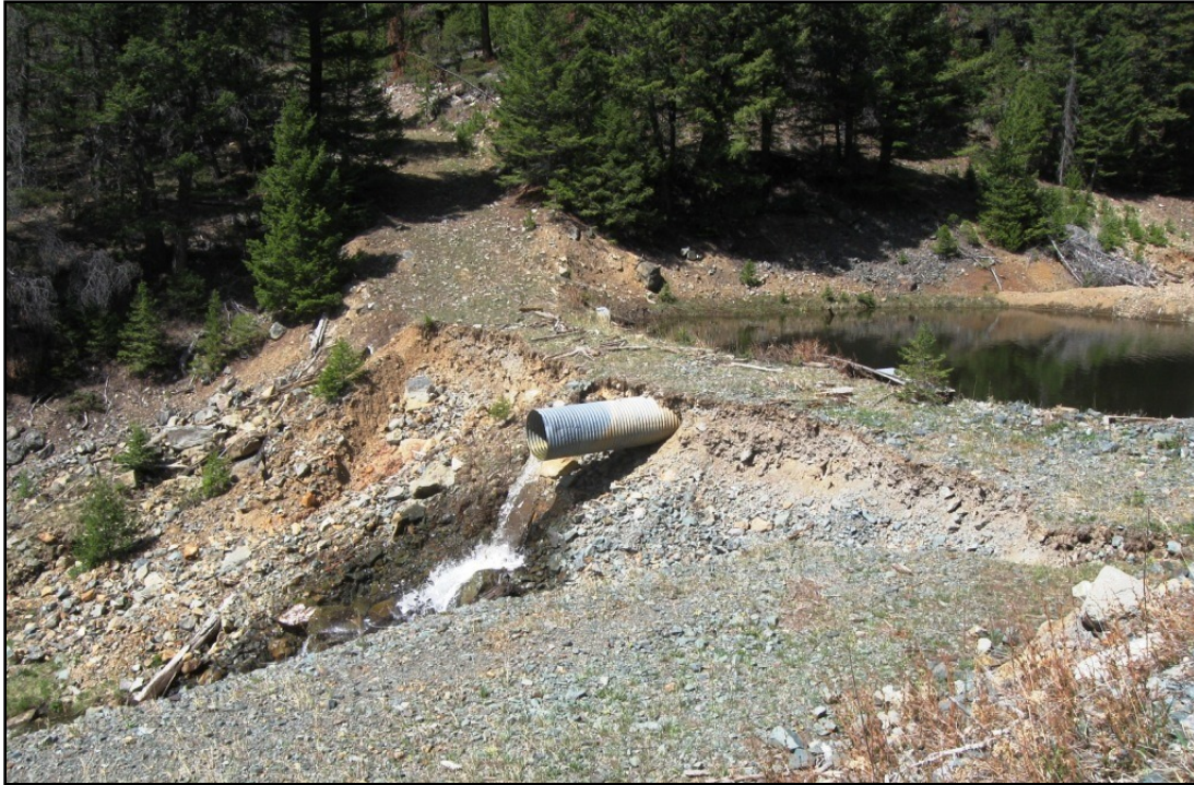
Erosion of dam impounding Indian Creek.
