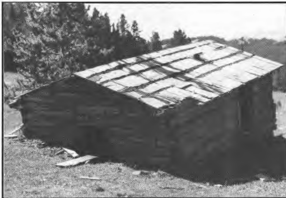
Figure 23. Rear and side of Feature 3 residence at northeast corner of 24BW210.
