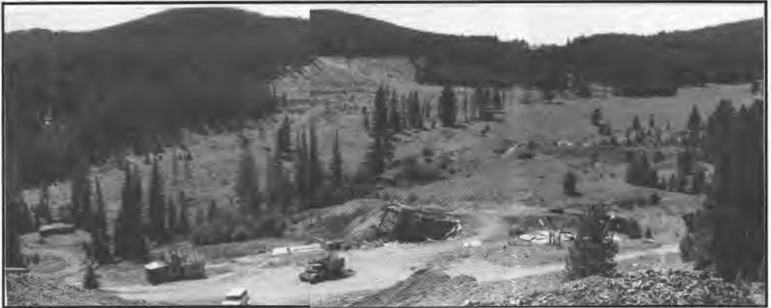
Figure 21. Panoramic view of west edge of 24BW210. Pictured features include Feature 62 residence (far left), Feature 63 assay office (next right), Feature 37 mill foundation (center), and Feature 69 dam (right).
