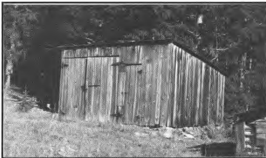
Figure 38. Feature 51 garage; shed addition on Feature 51 residence at right.
