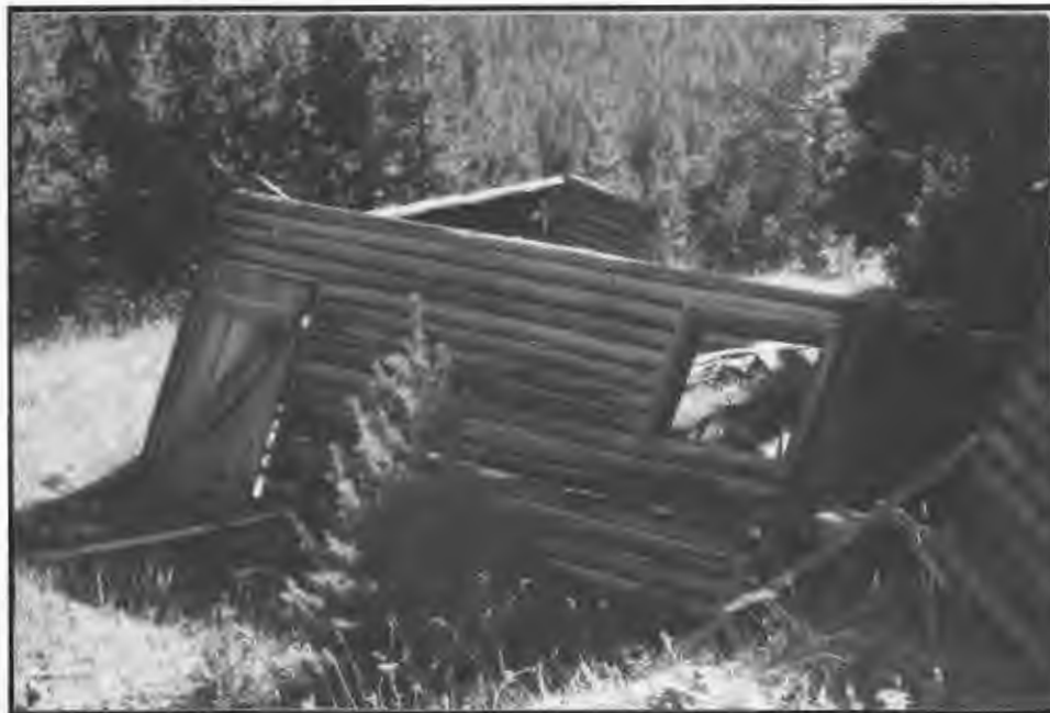
Figure 35. Partially collapsed Feature 17; Feature 16 outhouse at far right.
